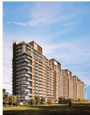
AG ATELIER GREENS KOREGAON PARK ANNEKE, PUNE.
